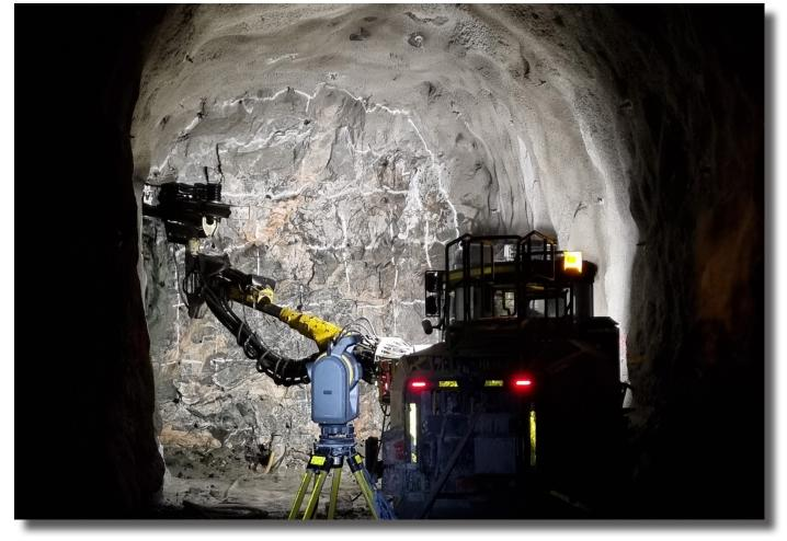
The integration of the digital cameras and removal of the telescope is a game changer for a one-man operation and allows for the highest level of efficiency for survey tasks.
